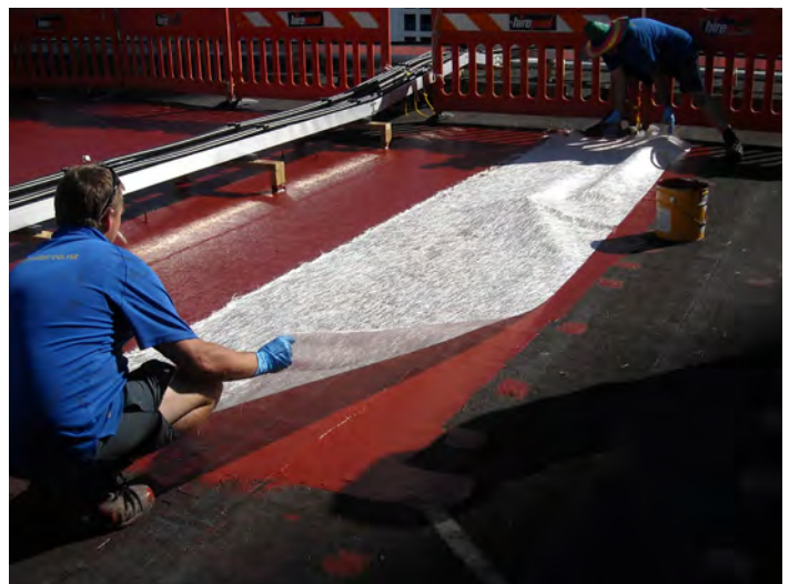
3. The reinforcing mat layer is rolled into the basecoat.
