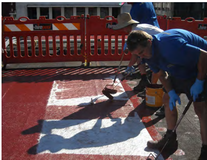
2. A reinforcing mat layer is added.
