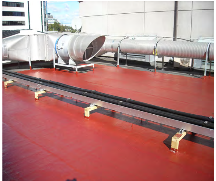
1. The standout red undercoat goes down.
