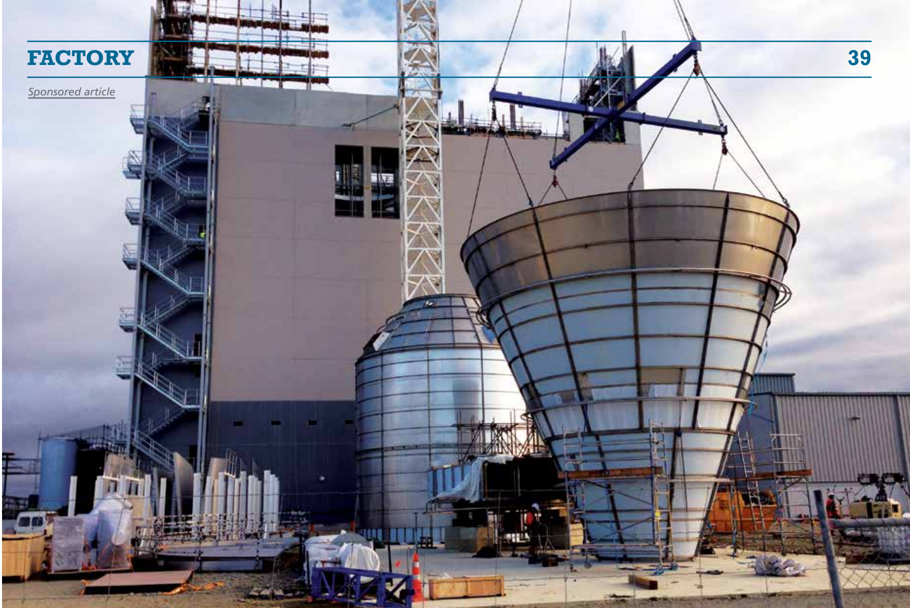
Oceania Dairy infant formula plant in Glenavy under construction
