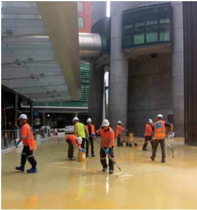
Sikafloor-375, Abrasion layer being applied at the Sky Hotel Entrance
