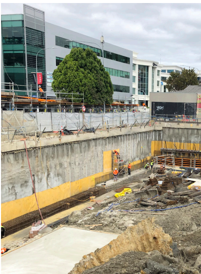
SikaProof Bentonite is a waterproofing system which efficiently protects reinforced concrete structures, preventing the penetration of water and subsequent attack by aggressive chemical substances present in the surrounding soil.
