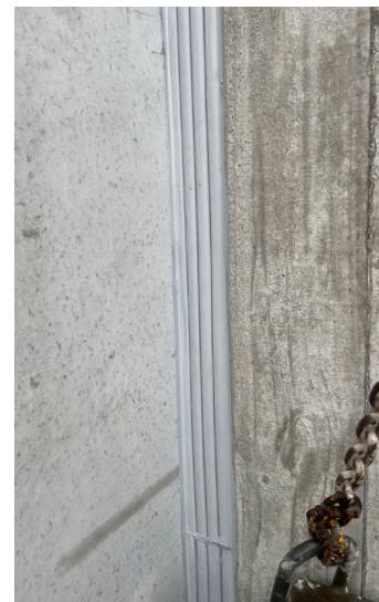
Seismic joints with Sika EMSEAL, a seismic joint system that is designed to provide both a watertight and trafficable joint sealing
