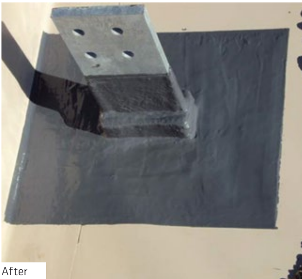
MEVAG AG BETTENWIESEN SWITZERLAND Various details of penetrations of steel columns.
