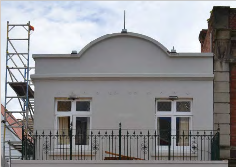
Figure 5: A strengthened heritage building, 280 Cuba Street, Wellington. (Photo: Wellington City Council, 2014)
