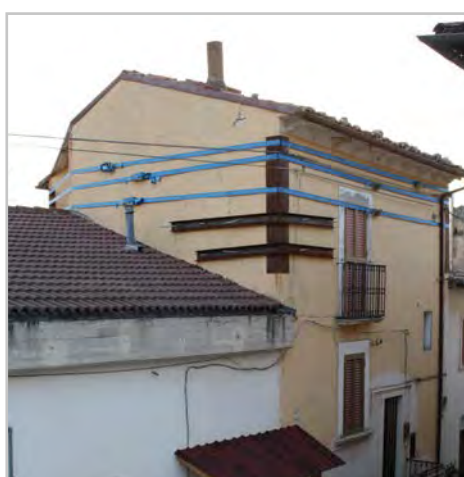
Figure 32: L'Aquila, Italy October 2011. Heavy-duty polyester webbing ratchet straps fitted around the building perimeter. Note steel angle plate to protect the straps, and distribute the clamping load into the corner masonry. (Photo: Win Clark)
