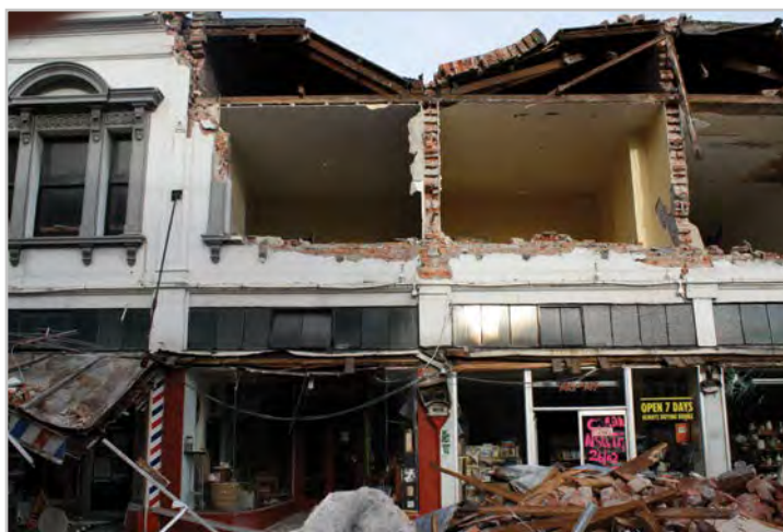
Figure 3: Christchurch, February 2011. Brick masonry parapet and facade have collapsed onto the pavement. Note only minor fixing between front facade brickwork and brick partitions at right angles. There is no fixing of facade brickwork back into roof framing that could provide support from the body of the building. The extension of the partition wall above the roofline has collapsed onto the adjacent roofing. Other areas of failure associated with facades are the brick piers between window and door openings, and brick masonry return walls adjacent to front facades. (Photo: Win Clark)
