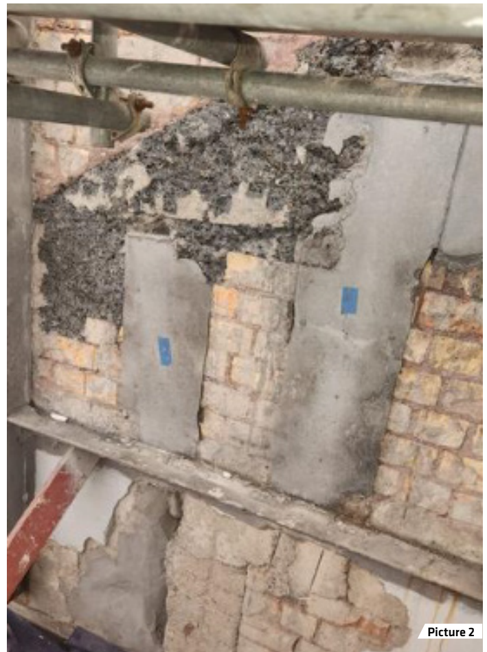
Picture 2: The repair was completed using Sika MonoTop®-438 R, with the formwork removed to reveal the reinstated concrete surface and restored structural profile.
