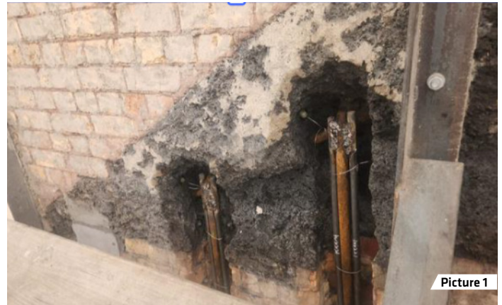
Picture 1: Deteriorated concrete was broken out to expose reinforcement, with Sika FerroGard® Patch anodes incorporated to help prevent future corrosion.
