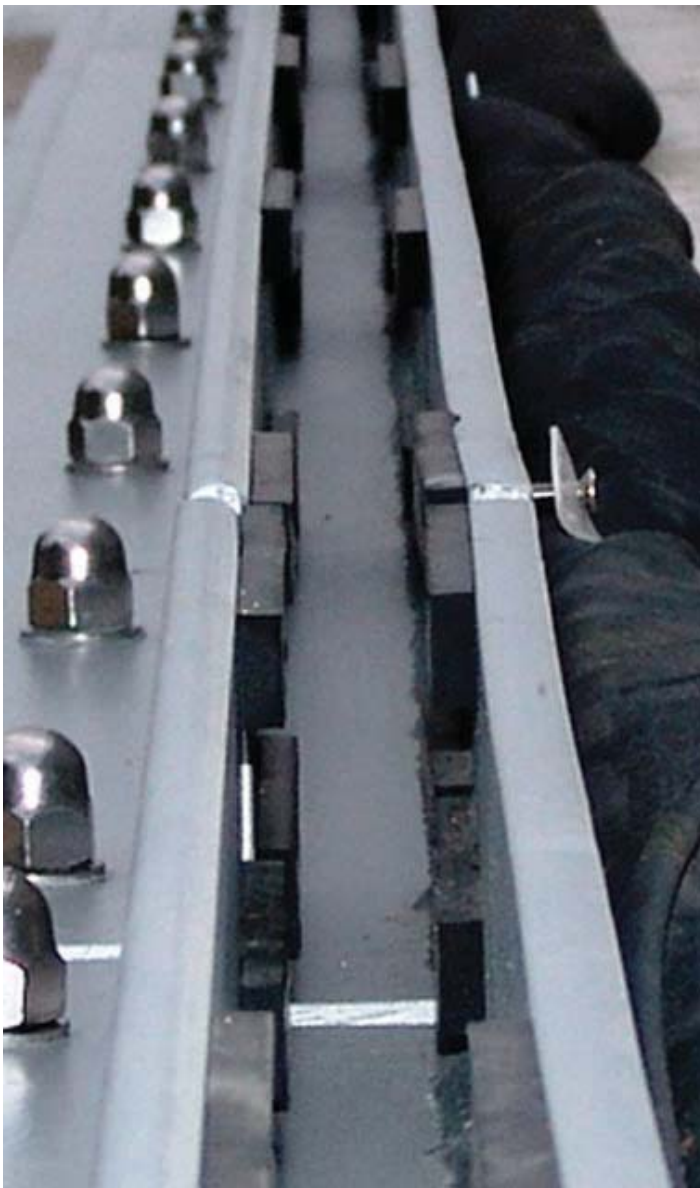
Picture 5: Glass fixing blocks in U-channel
