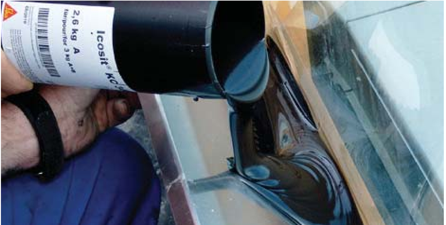
Picture 12: Pouring of Sika Icosit KC 340-7
