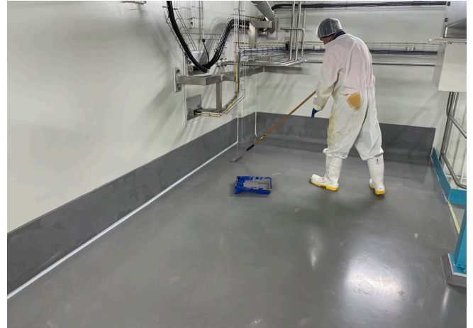
Sikafloor-21 PurCem smooth finish, grey, being applied to dry areas.
