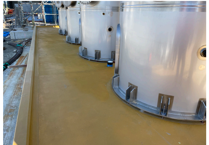
Sikafloor PurCem non-slip screed, maize yellow, to exterior silo areas.
