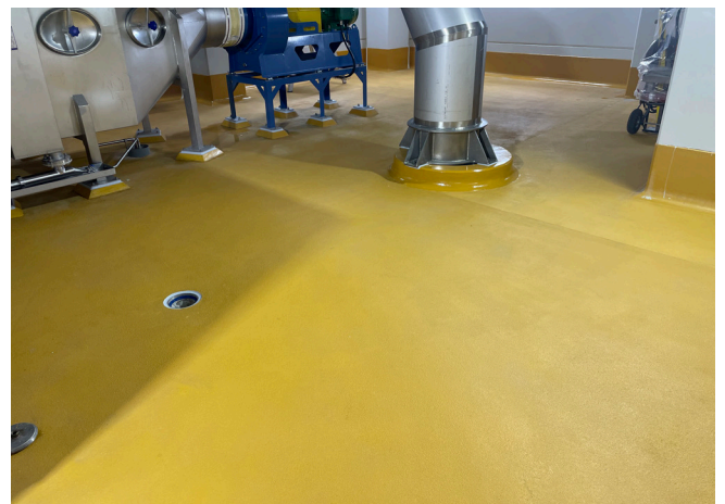
Sikafloor PurCem non-slip screed, maize yellow, to interior processing areas.
