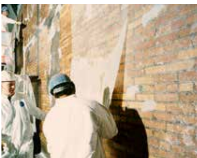
SEISMIC UPGRADING /EARTHQUAKE DAMAGE REPAIR
