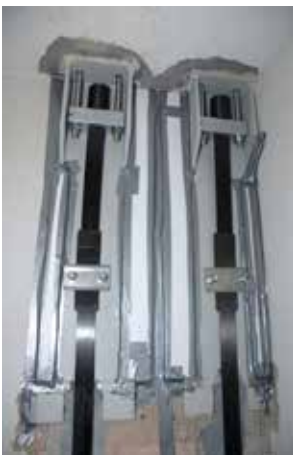
Anchorage of Sika CarboStress System
