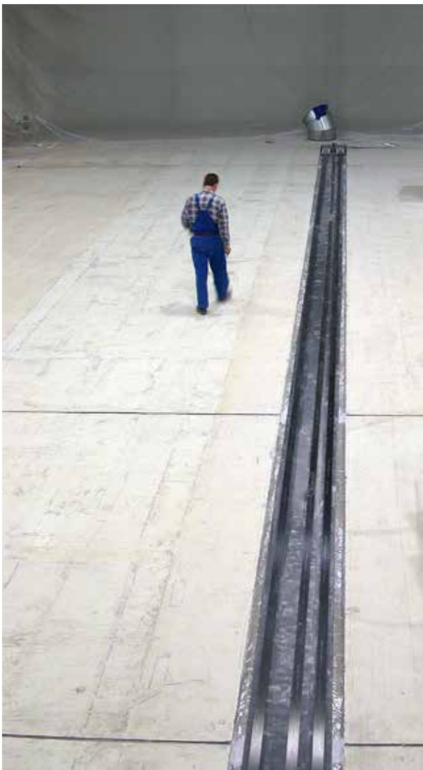
The longest post-tensioned CFRP-plates ever installed
