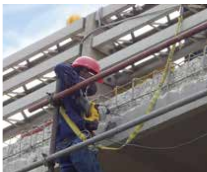
Substrate preparation
