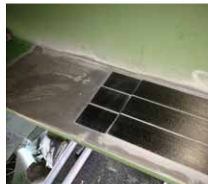
Two layers of Sika CarboDur®
