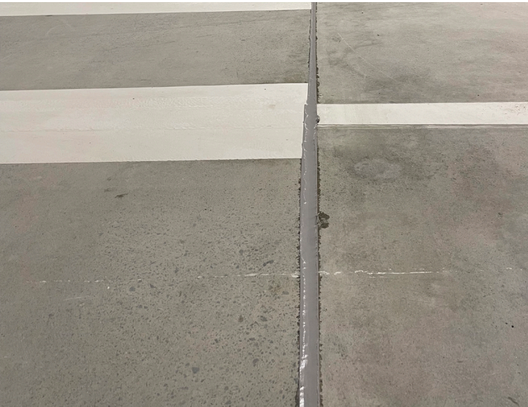
Completed photo: Sikaflex® PRO-3 Purform®, polyurethane sealant for floor joints in civil engineering structures
