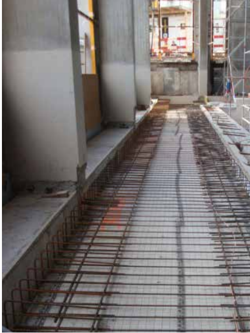
Reinforcement of the the swimming pool surrounding.
