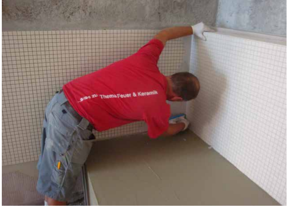
Grouting of the stoneware mosaic with SikaCeram®-EpoxyGrout
