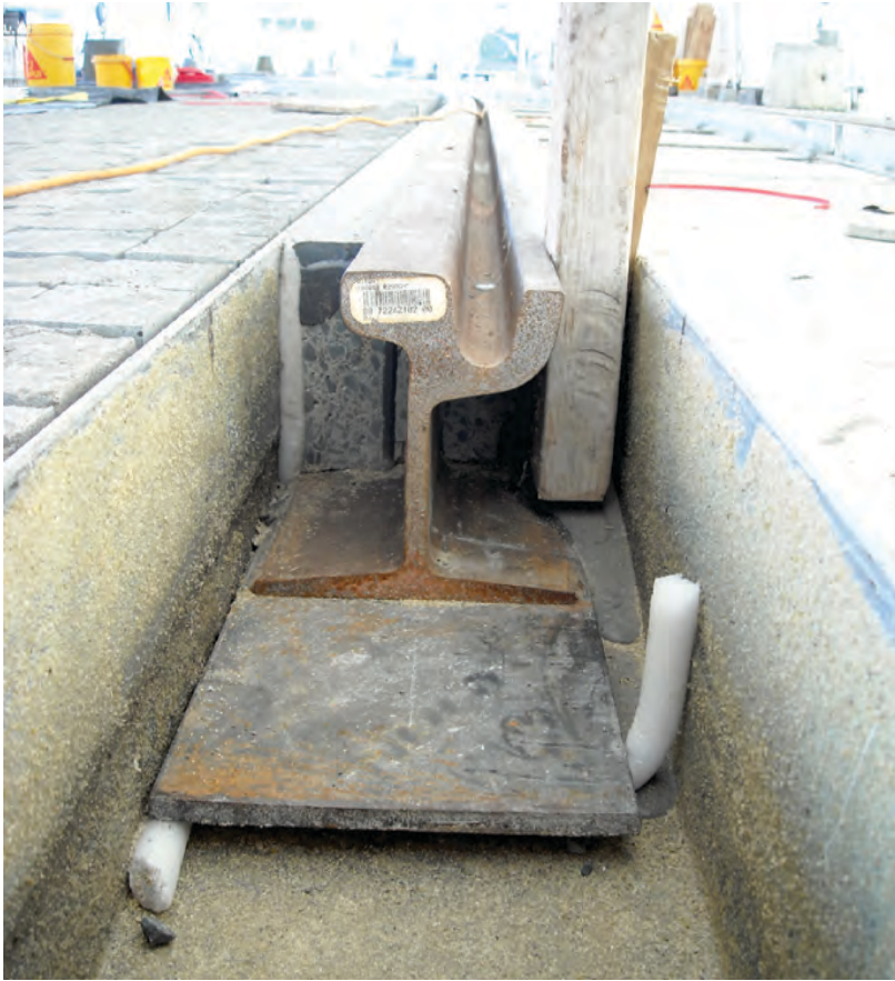
SIKA'S ICOSIT RAIL BONDING SYSTEM solved three major challenges for the new tram loop around the Wynyard Quarter on Auckland's waterfront
