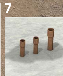
Leaking Penetrations i.e. Pipe Penetrations
