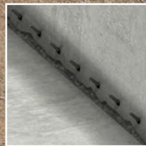
Leaking Construction Joints
