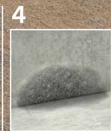
Leaking Areas of Voids i.e. Honeycombing
