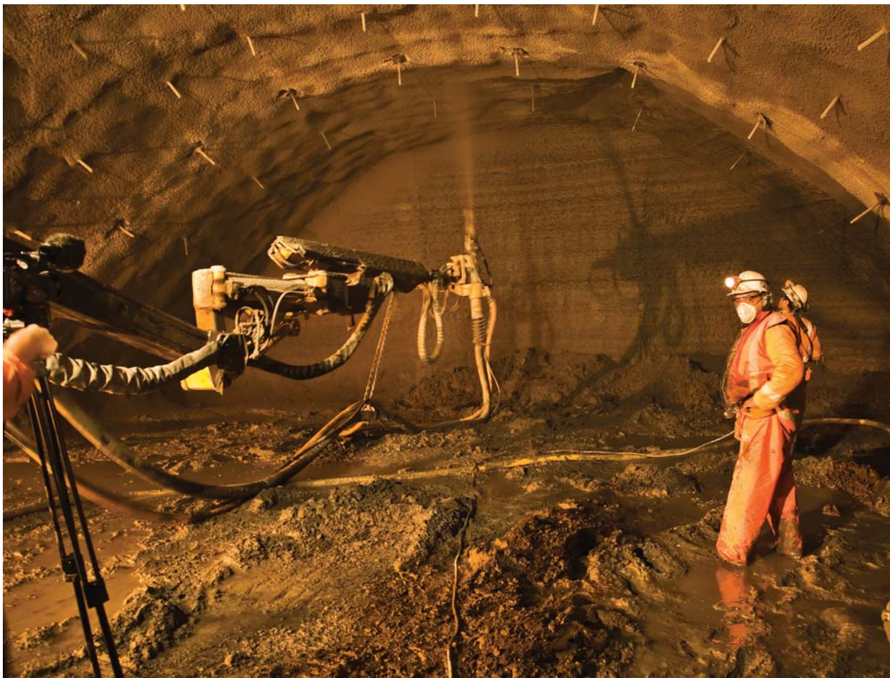
The Sika Aliva PM500 robotic arm sprays the shotcrete containing Sika ViscoCrete SC305 retarding superplasticiser, and Sigunite L53-AF accelerator for sprayed concrete
