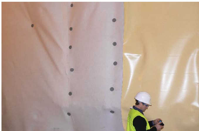
Sikaplan FPO being applied over felt protection material
