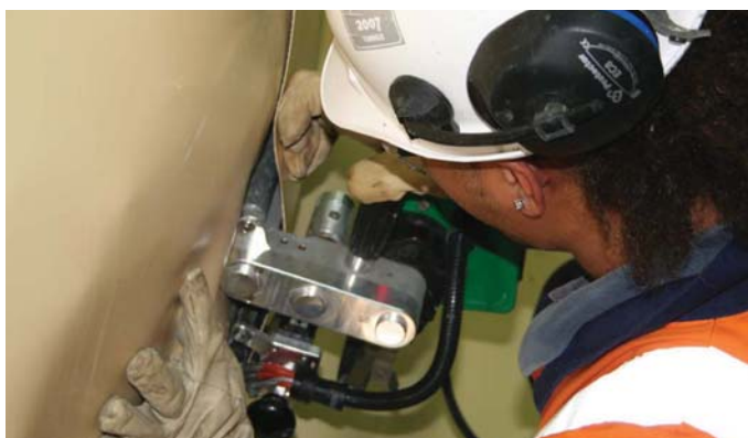
Application of the Sikaplan FPO in the tunnel
