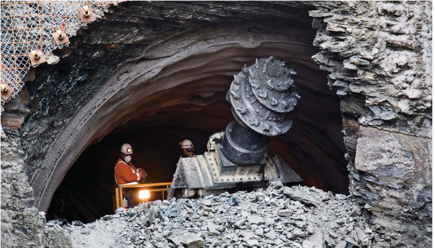
Breaking through to the otherside of Johnstone's Hill
