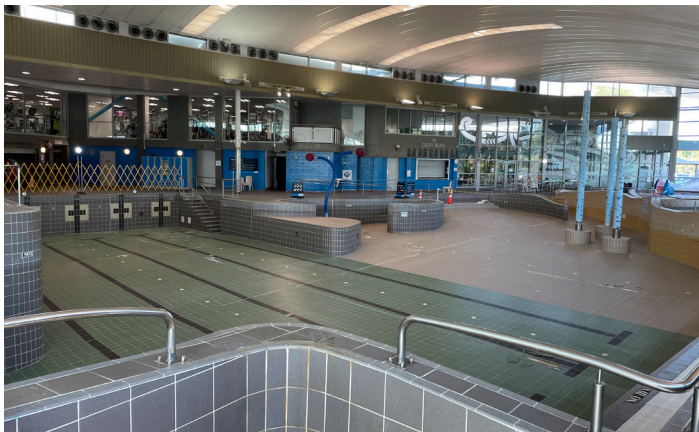
Before: Pool was drained to inspect the condition of the joint.
