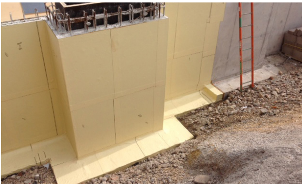
Open excavation with protrusion slab to wall: The complete structure is sealed with SikaProof® P.
