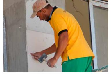
SikaCeram®-205 Large: Cementitious tile adhesive consisting of high quality cements, selected silica/quartz sands and specific additives with a high polymer content. It is suitable for installing tiles on building facades and for outdoor use.
