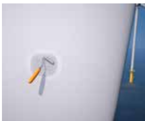
Spreading of resin.
