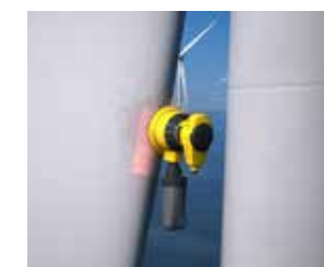
Sanding of repaired area.
