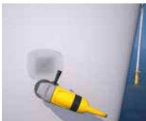
Chamfering of damaged area.
