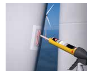
Application of SikaForce®-7800 on prepared surface.
