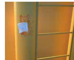
Cleaning of damaged surface.
