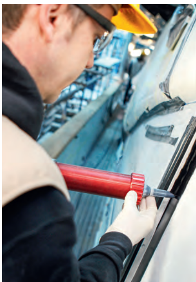
Fig. 6 Adhesive is applied to the window frame
