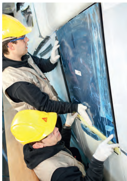
Fig. 7 The window is fitted
