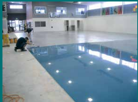
A self-smoothing layer of seamless Pulastic floor is then applied.
