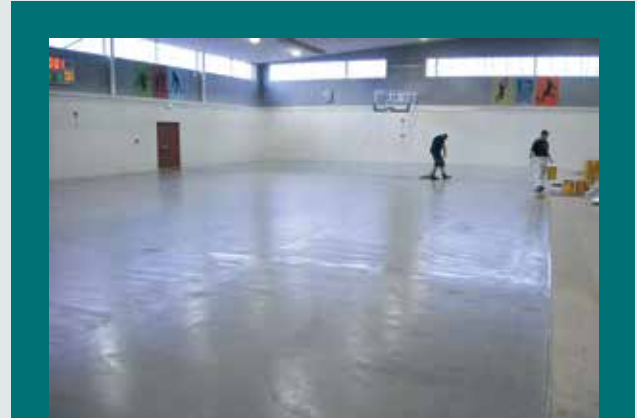
A 2mm base layer is applied on top of a 7mm shock absorbing mat.
