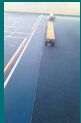
A self-smoothing layer of seamless Pulastic floor is then applied.
