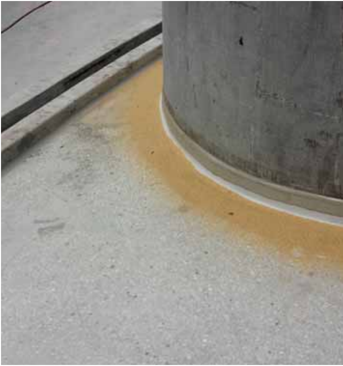
Sikadur Combiflex SG used on the Sky Tower pillars / columns
