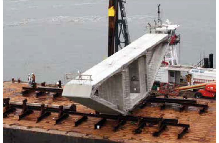
The precast element shipped to building site
