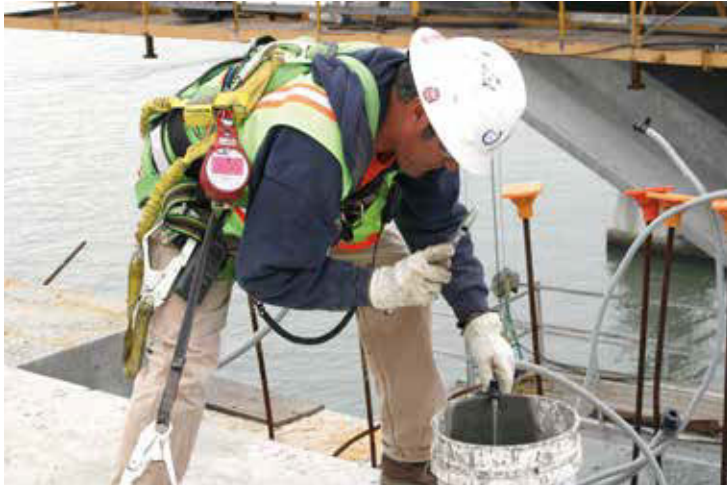
Grout coming out of the air pipe
