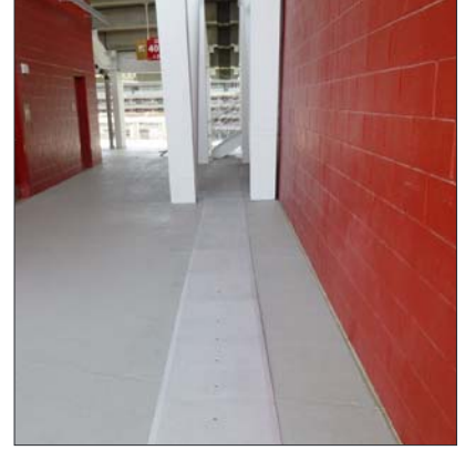
Concourse Joints Split or Solid Slab
