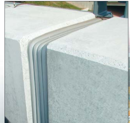
Vertical Plane Structural Separations: Parapet & Transitions
