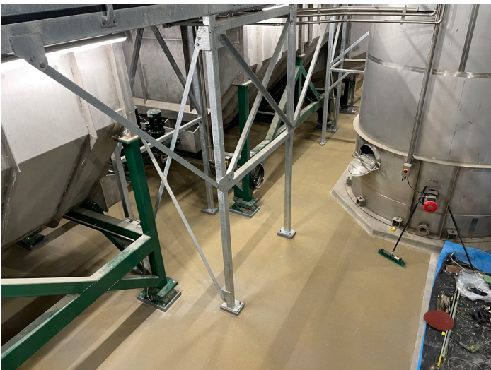
Above and Below image: Sikafloor® PurCem® high performance floor screed installation completed.
