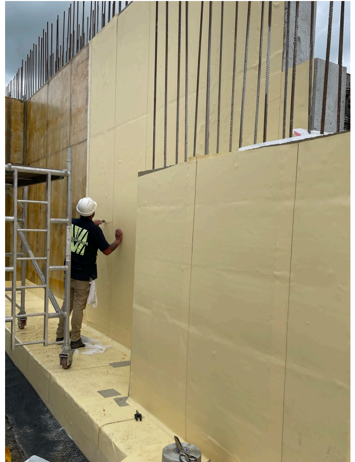
SikaProof® P-12 self-adhesive sheet membrane - shows the height of the significant basement prior to backfilling.
