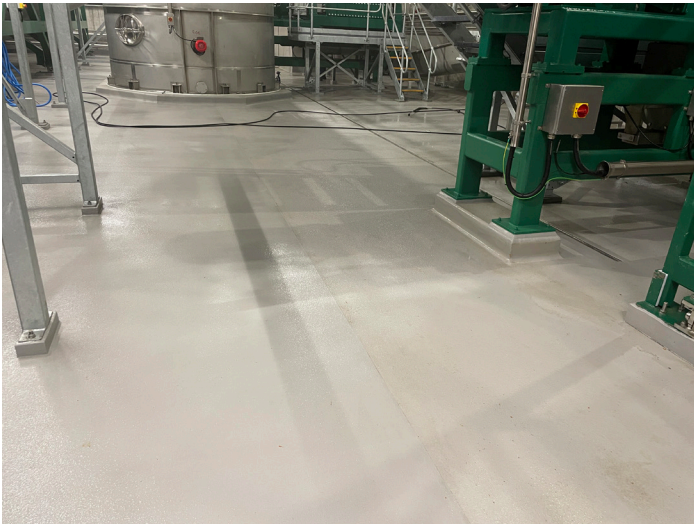
Above and Below image: Sikafloor® PurCem® high performance floor screed installation completed.
