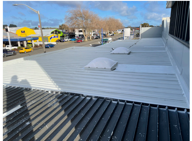
During coating stage
