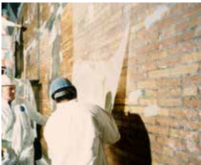
SEISMIC UPGRADING /EARTHQUAKE DAMAGE REPAIR
