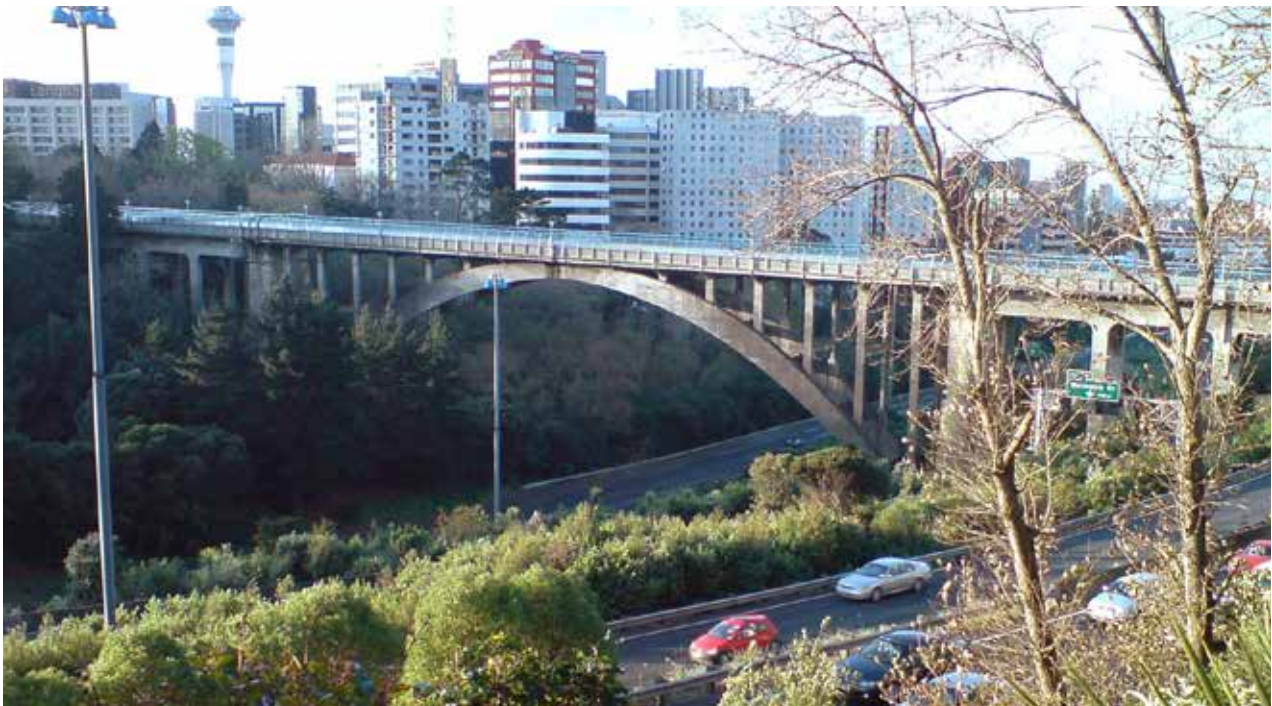
Grafton Bridge, Auckland, New Zealand
