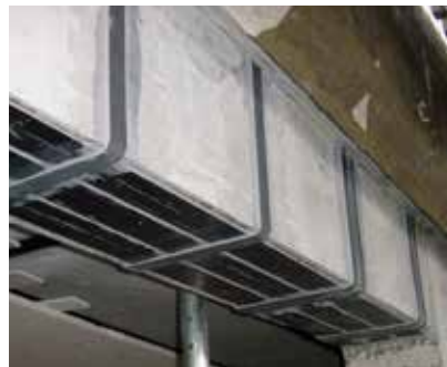
BEAM STRENGTHENING
