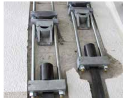
PRE-STRESSED STRENGTHENING
