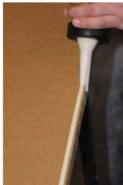
Apply bead to seal joints.
