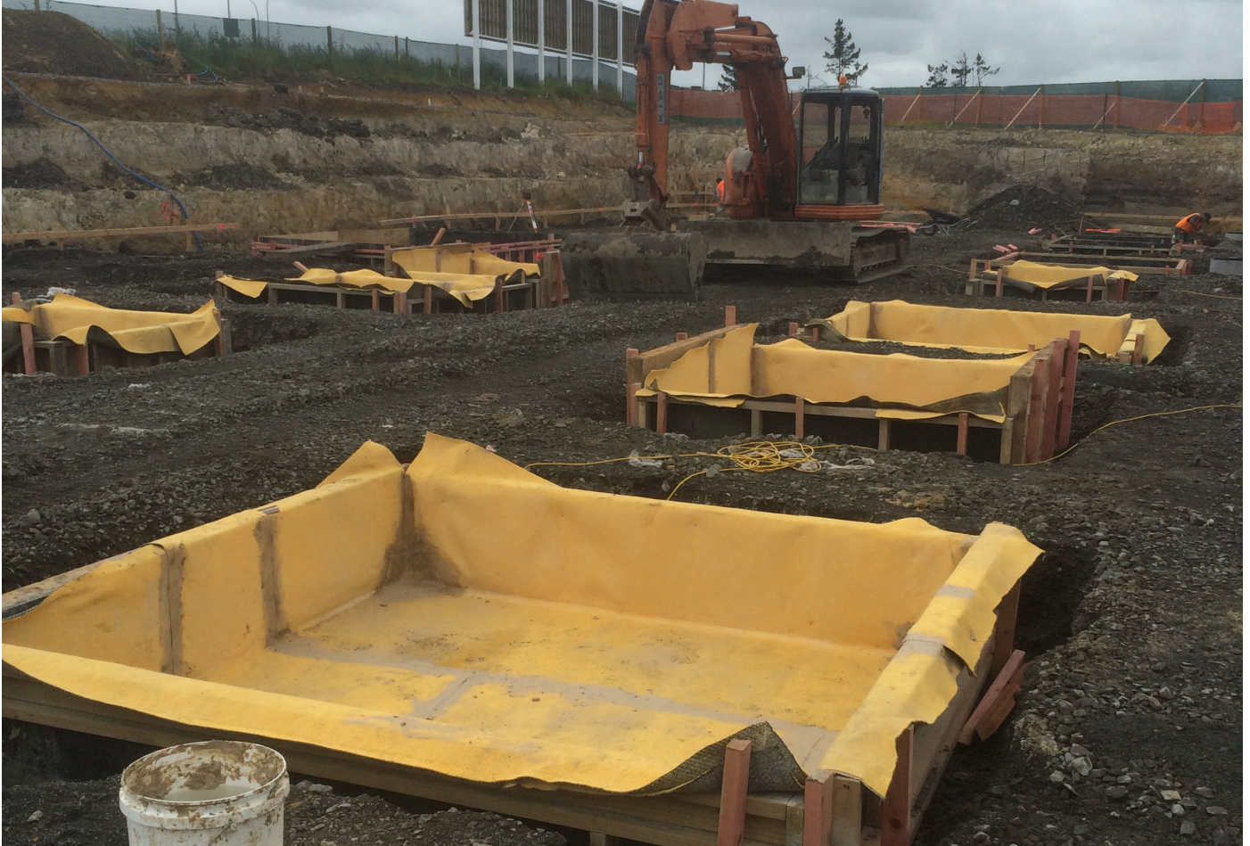
Waterproofing of pad foundations for basement slab
