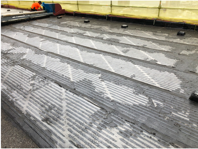
Sika Index Tectene BV Strip Vapour Barrier strip over insulation
