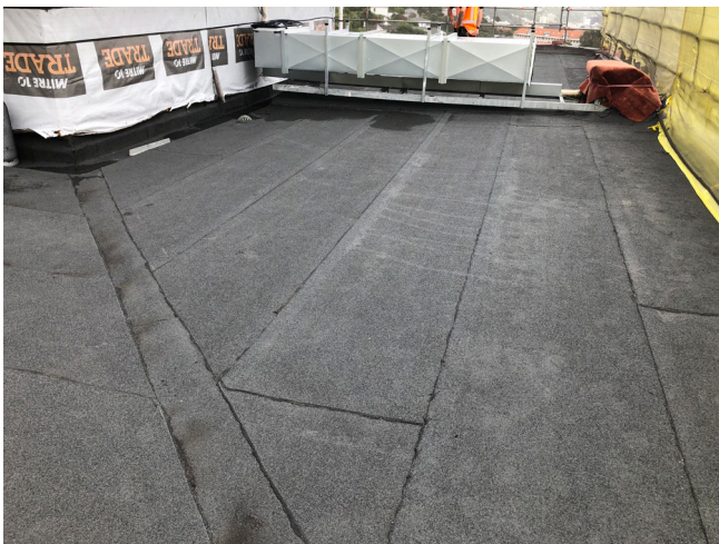
Sika Index Mineral Proteaduo Triarmato cap sheet over the BV strip
