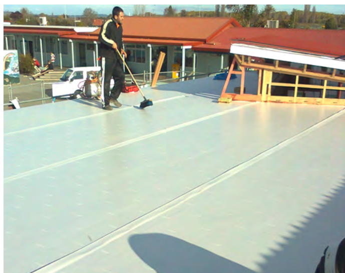
Gunac Hawkes Bay install the fully-adhered Sarnafil roofing membrane system at Arthur Miller School.
