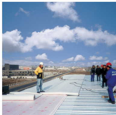
Lightweight Roof (Nokia Plant, Beijing, China)
