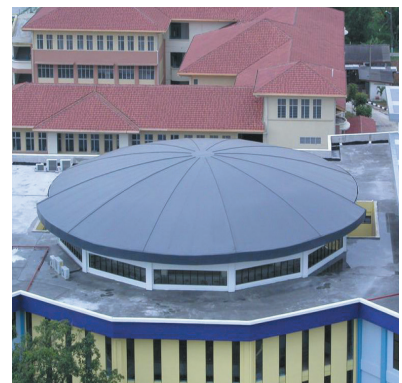
Exposed Roof (Sentul School, Malaysia)
