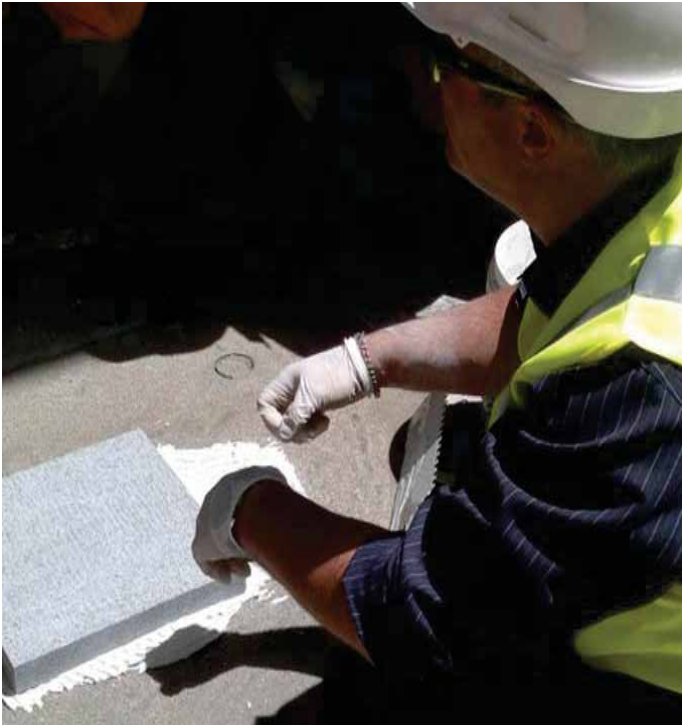
Direct tile bonding to Carpark Deck System broadcast to excess
