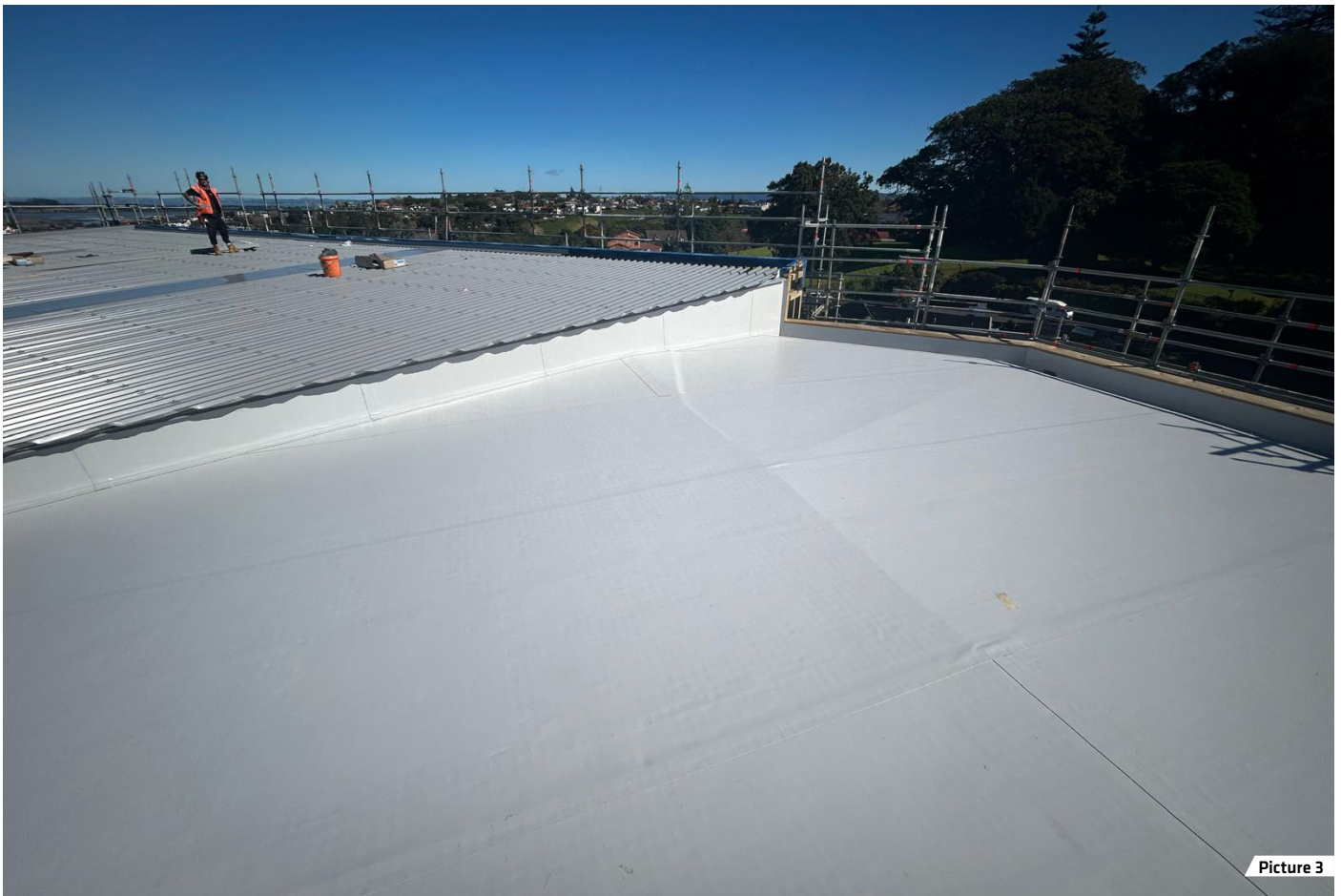
Picture 3: Sarnafil® roofing membrane successfully installed to the Level 6 roof area.
