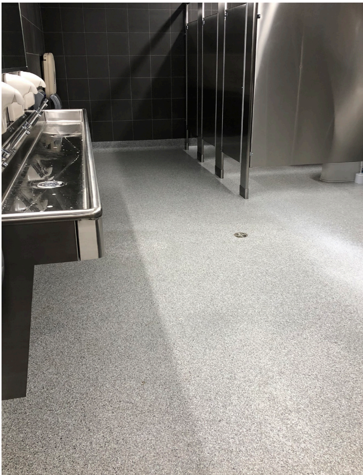
Sikafloor ® -264 (Vinyl Chip Flake 'Richmond Marble') - Toilet facilities
