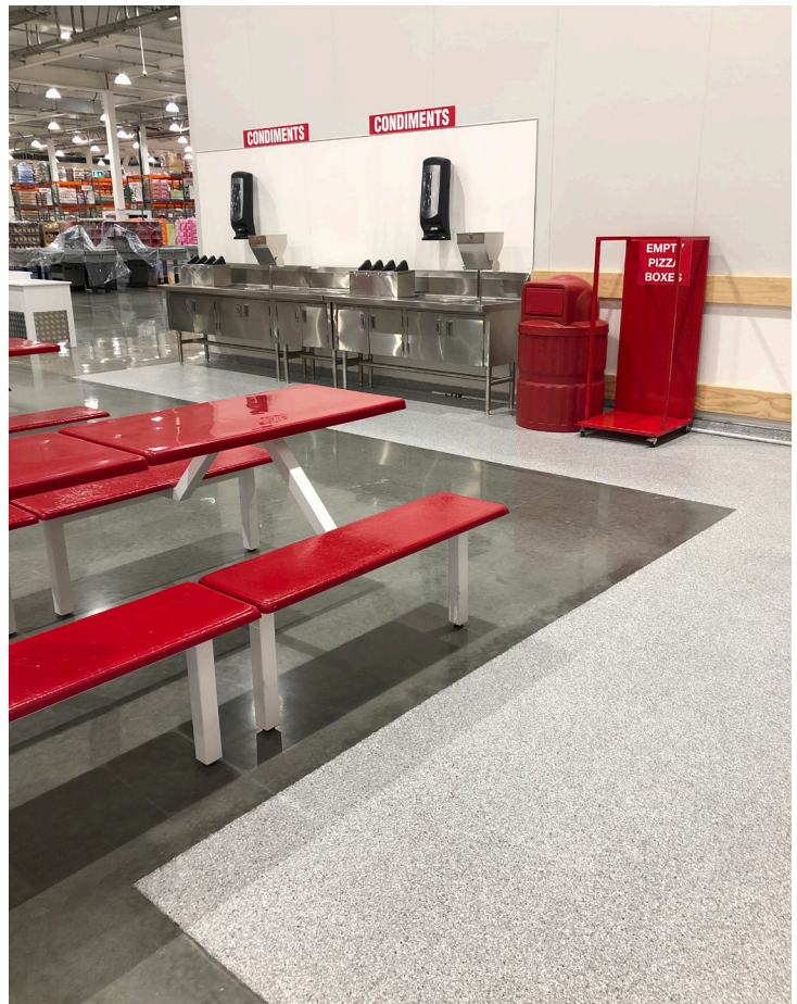
Sikafloor ® -264 (Vinyl Chip Flake 'Richmond Marble') - Bakery and Kitchen Areas
