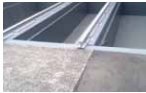
Solutions for Secondary Containment Areas. Page 20
