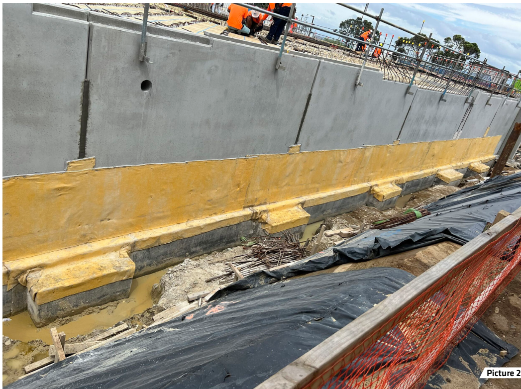
Picture 2: SikaProof® Bentonite installed over pre-cast concrete panels
