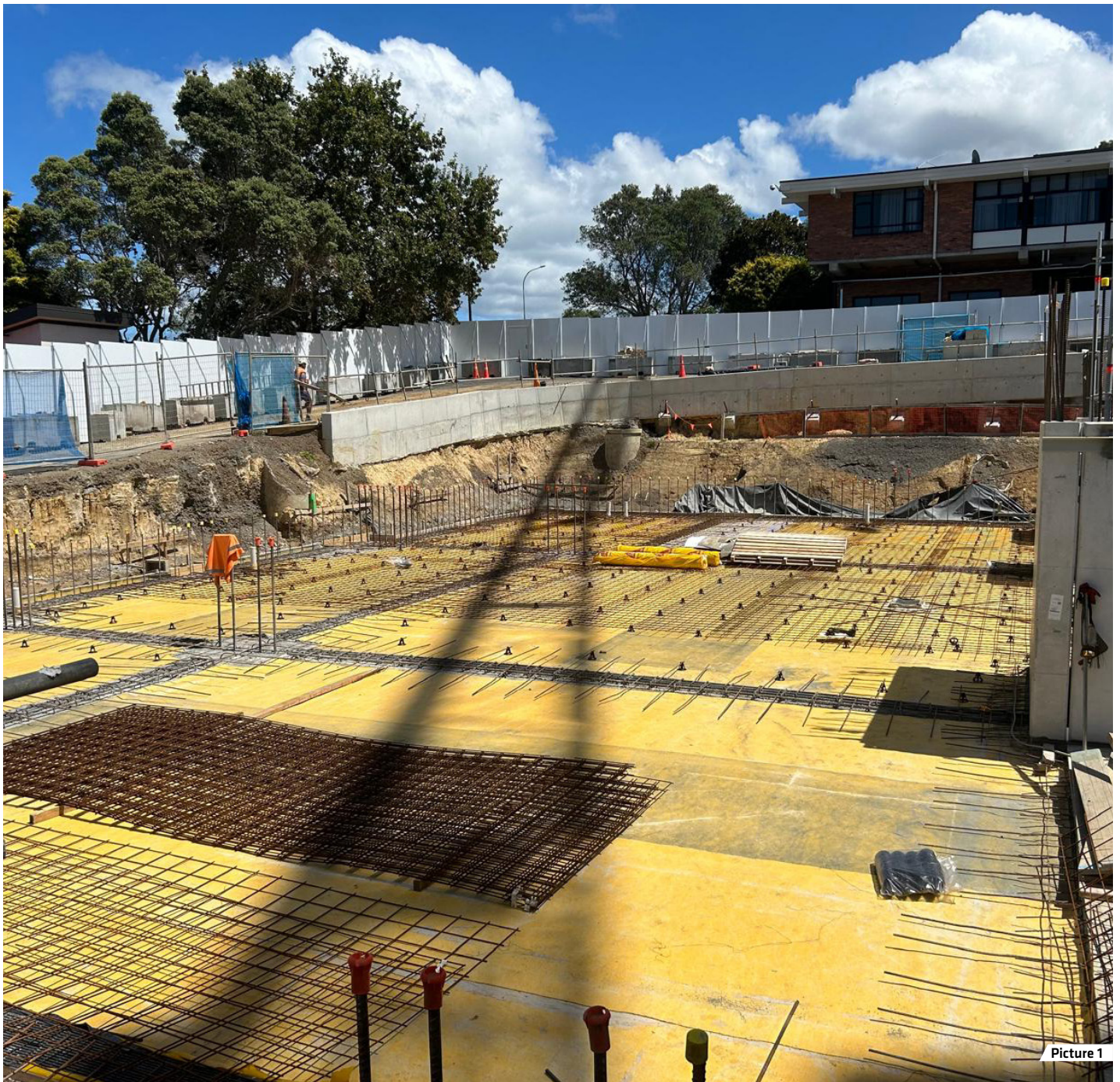
Picture 1: SikaProof® Bentonite has been installed prior to the basement slab pour.
