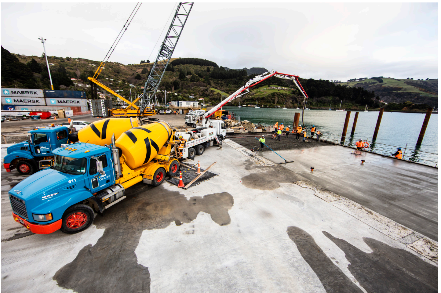
All photos courtesy of Allied Concrete
