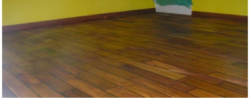
New wood floor installed by bonding over the old existing tiles, then caulked like a boat deck with Sikaflex®-290 DC.
