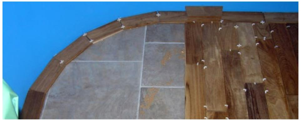
Easy renovation with SikaBond adhesives bonding the new wooden floors directly on the old existing tiles.
