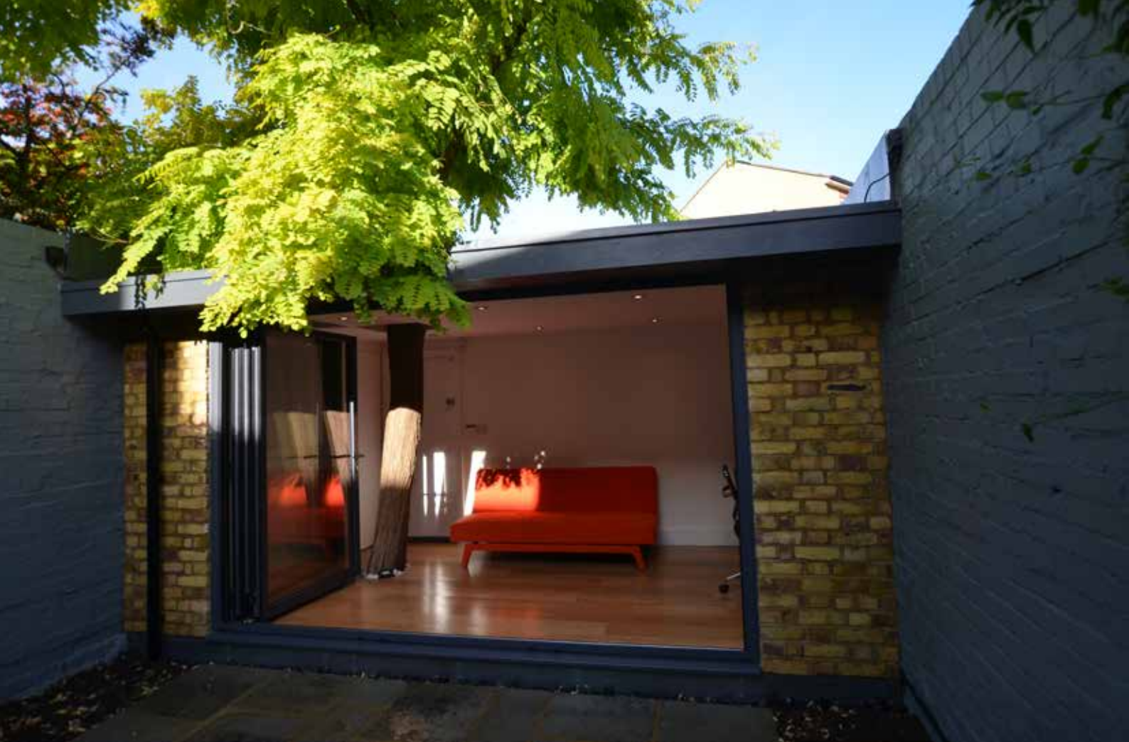
The garden room, designed by Leckenby Architecture, in Hackney. Sika Sarnafil's durable and flexible single ply membrane was used in the roof to allow the tree to grow and sway.
