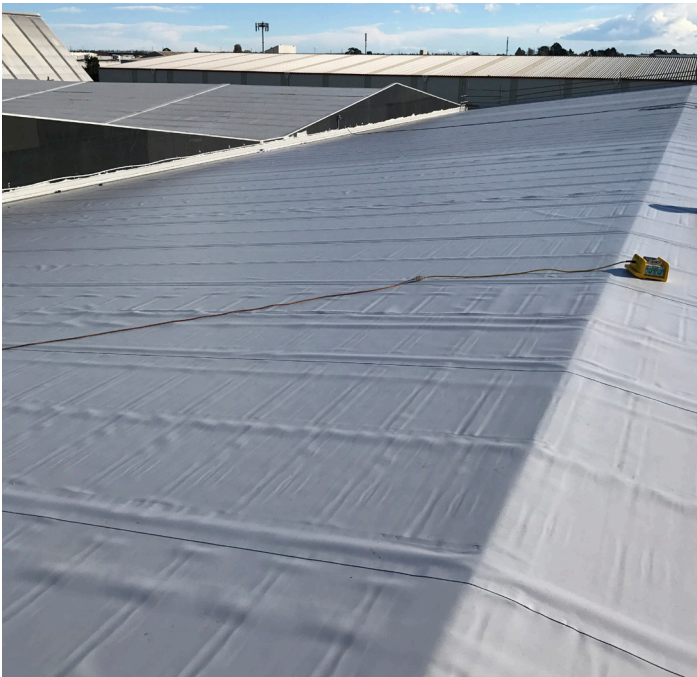
After: Sarnafil S 327-20 L installed over existing roof
