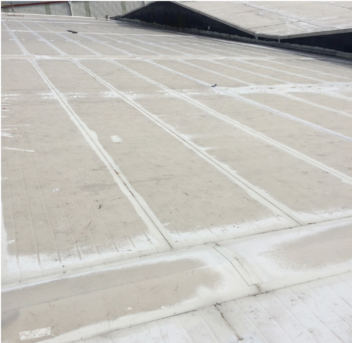
Before: Existing freezer roof
