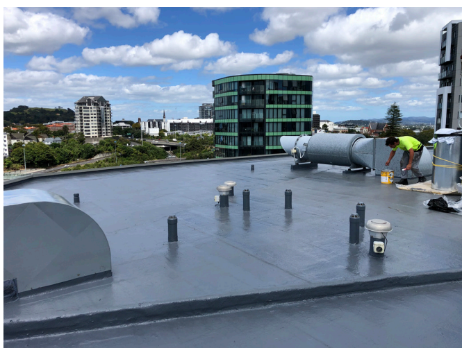
Finished system of SikaRoof MTC (now i-Cure)
