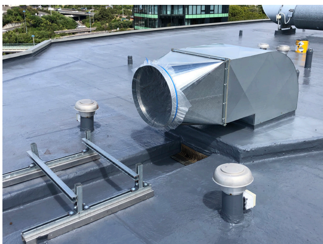
Penetration detailing - no problems for SikaRoof MTC (now i-Cure)
