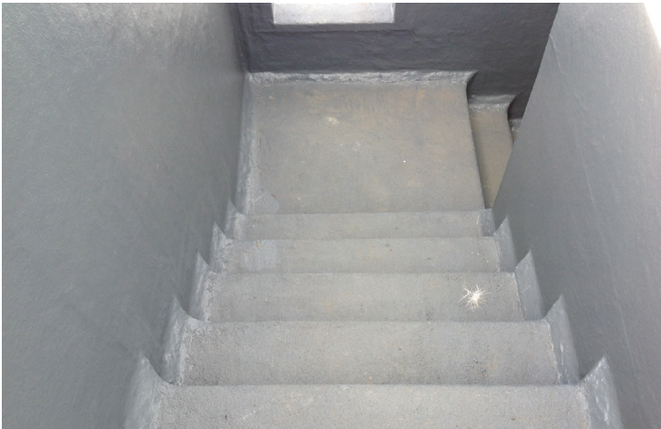
Sikalastic-621 TC, part of the SikaRoof MTC System has been used to waterproof the stairwell.
