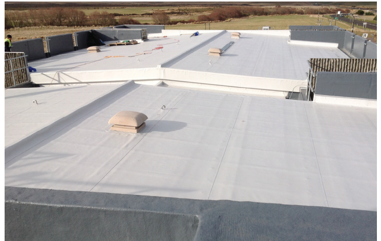
Sarnafil and SikaRoof MTC systems on the Museum's roof.
