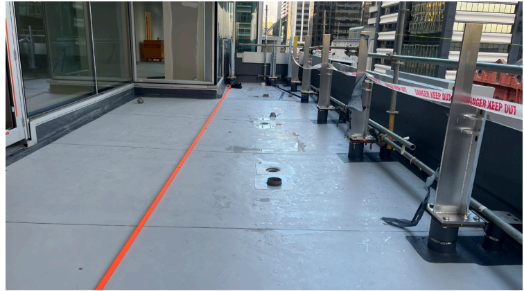
Sika Sarnafil membrane provides reliable and durable waterproofing to areas being concealed with pavers on pedestals. The use of sacrificial pads of Sika Sarnafil above the main membrane assists in isolating direct contact from the pedestals themselves.
