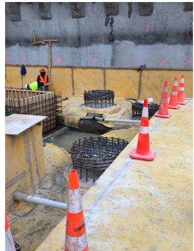
Using a combination of Sika accessories, such as pre-formed corners and PVC membrane-laminated metal sheet, detailing can be simplified and robust, complimenting Sika Sarnafil's reputation for decades of durability.
