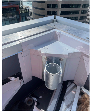
Using a combination of Sika accessories, such as pre-formed corners and PVC membrane-laminated metal sheet, detailing can be simplified and robust, complimenting Sika Sarnafil's reputation for decades of durability.
