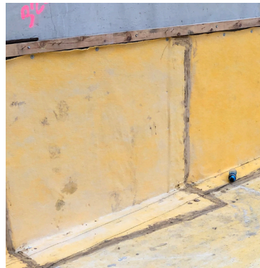
SikaProof Bentonite is a waterproofing system which efficiently protects reinforced concrete structures, preventing the penetration of water and subsequent attack by aggressive chemical substances present in the surrounding soil.
