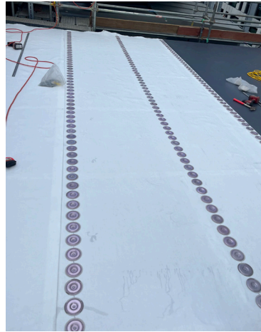
Sarnaweld Discs are attached directly to the substrate, and these PVC-coated plates are then induction-welded to the underside of the Sika Sarnafil membrane.
