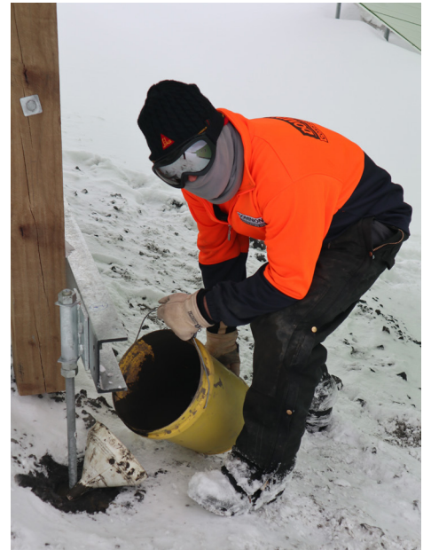
All photos courtesy of Dominion Constructors Ltd
