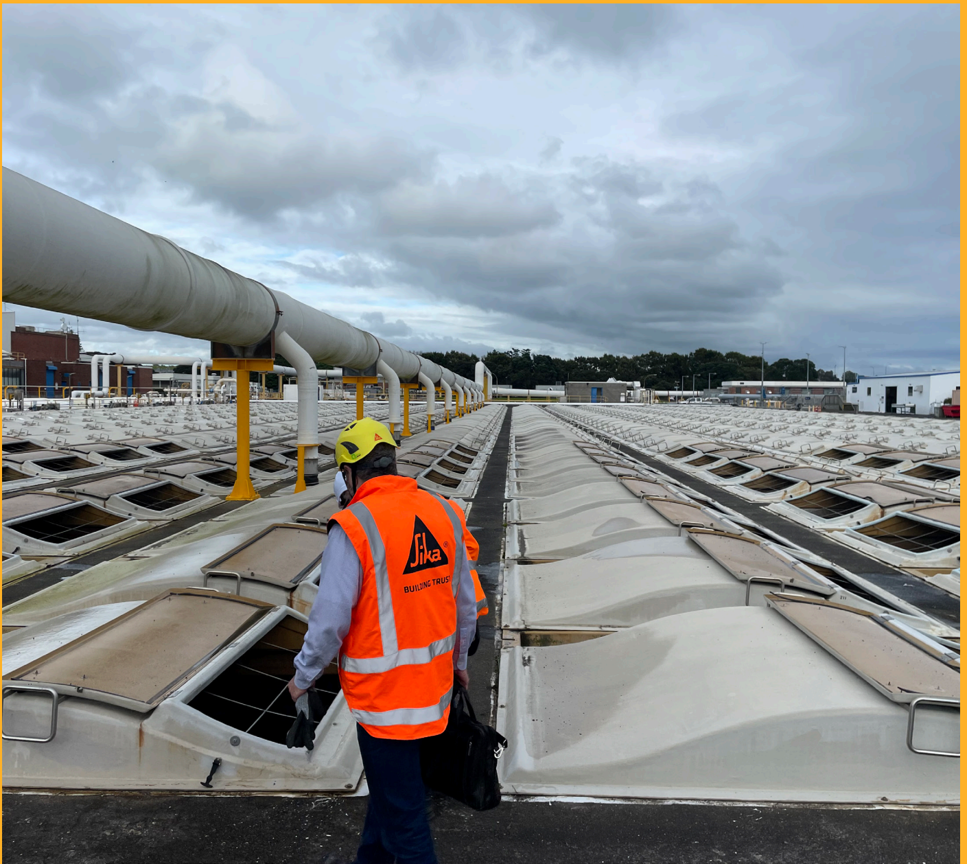
Mangere Wastewater Treatment Plant, Auckland
