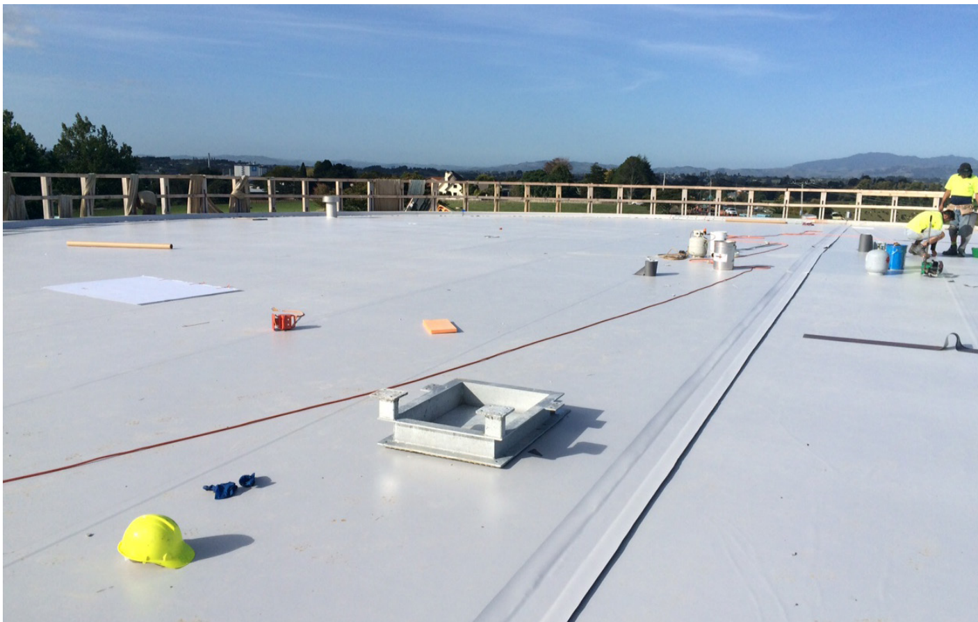
Contractor, Arid Technologies Ltd work on final stages of the roof membrane installation
