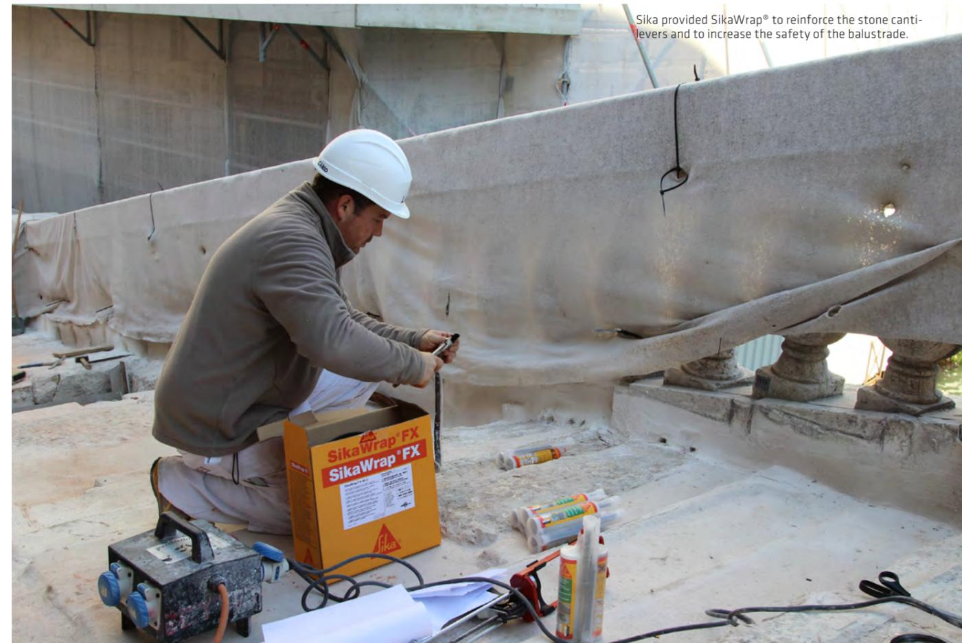
Sika provided SikaWrap® to reinforce the stone cantilevers and to increase the safety of the balustrade.
