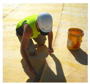
Watertight the Waterproofing People Ltd installed 7,000m<sup>2</sup> of SikaProof Bentonite
