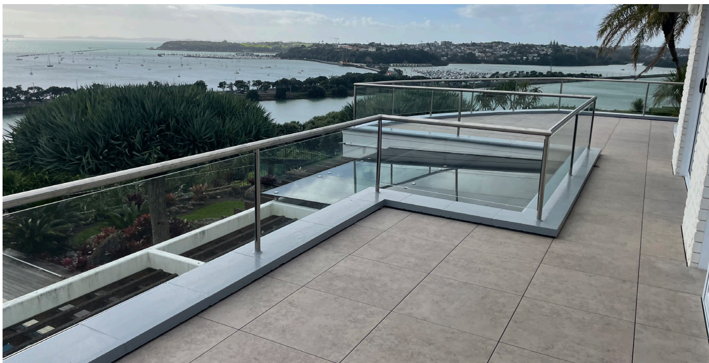
Finished deck with tiling on pedestals over the SikaRoof® i-Cure-22 system.
